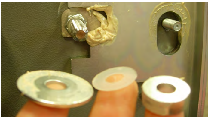
Top C: Handle Spindle with Cam & Locknut Bottom L to R: Guide Flatwasher, Nylon Washer, Bushing
